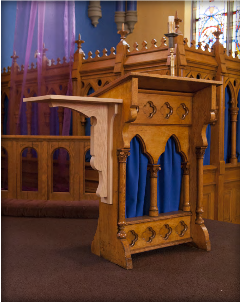
Installed before finish matching.
